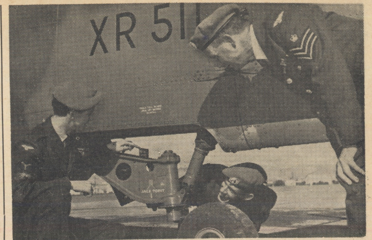
ABOVE: 18 Squadron ground crew inspecting the tail wheel assembly on a Wessex helicopter. LEFT TO RIGHT: SAC Howard, SAC Chapman, Flight Sergeant Evans. BELOW: Checking over the main rotor assembly on one of the Squadron's helicopters are, LEFT TO RIGHT, Cpl Young, Sgt Mitchel, SAC Gooderham and SAC Stead.
