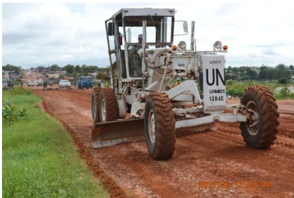
UNMISS Bangladesh Engineers using motor graders at work in Juba
