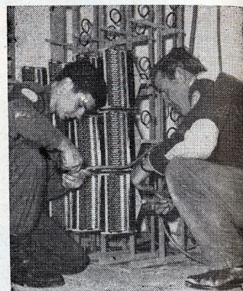
● Busily engrossed in the task of wiring the frame for the new telephone exchange are (left to right) Corporal Rick Francis, Canadian Signals, and Lance Corporal Ginge Stacey.
