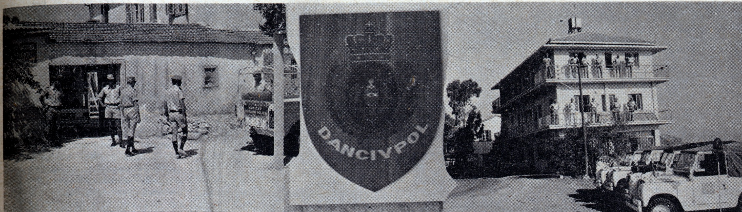
● The Danish substation in Ayios Theodoros — Entrance to Mess House, Camp Kronborg — Substation Dansborg, Xeros.
